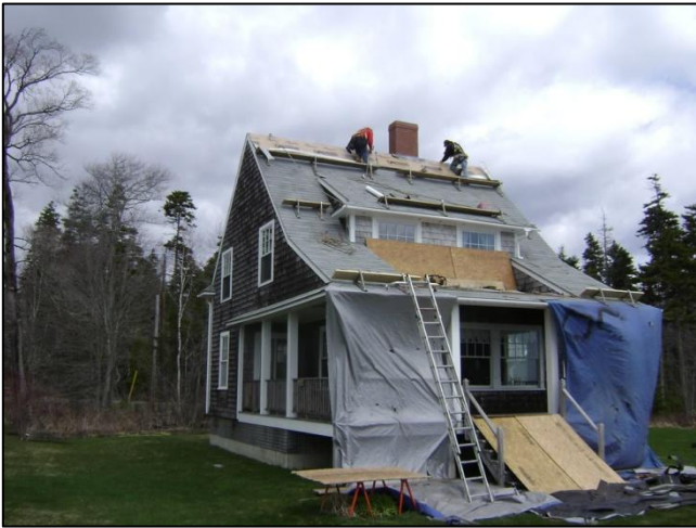
Waterproof Underlayment Secured
