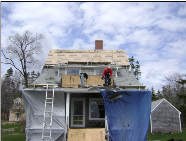
Crew Carefully Removes Roof Debris
