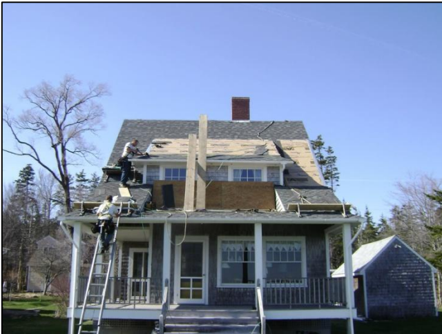
Crew Wears Safety Harnesses
