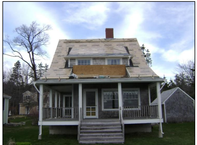
Debris Removed & Roof Weathertight
