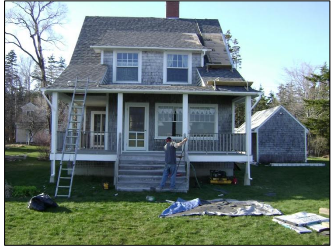
No Nails or Debris Left Behind
