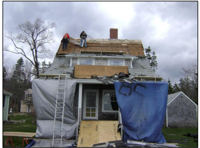
Rainproofing Stripped Roof Sections
