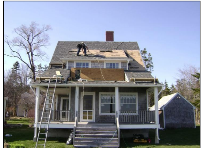
Roof Almost Finished
