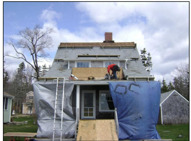
Shingle Stripping Begins at Peak
