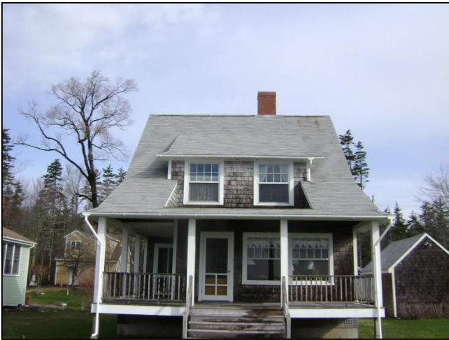
House Awaiting New Roof
