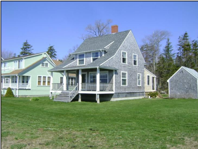
Finished Roof – Architectural Shingles
