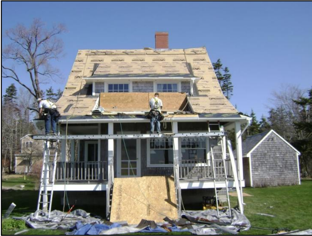
Ice & Water Shield on Eaves
